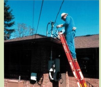
Don't take unnecessary risks with your safety! Arc-flash burns and other serious injuries can occur when working along energized service drops or other exposed electrical conductors.
